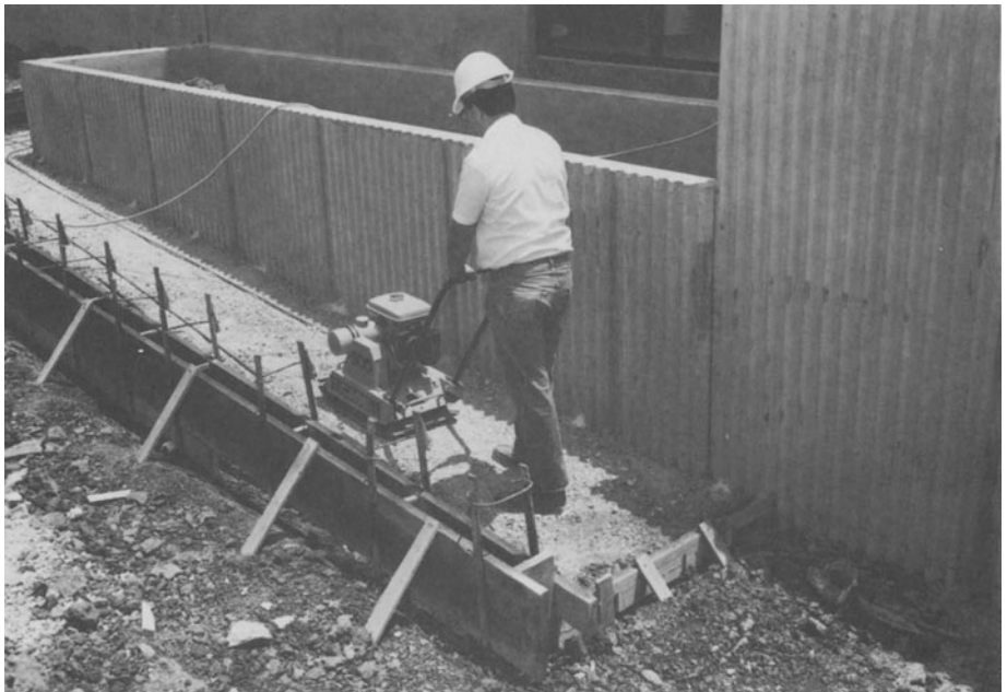
FIGURE 10-4. Different types of hand operated vibratory compactors. (a) rammer, (b) self-propelled plate compactor. [Ref. 7]
