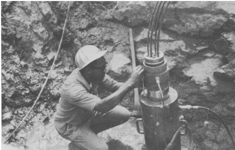
FIGURE 8-21. Measuring the rock anchor elongation after the cable has been pre-stressed. [Refs. 9 and 12]
