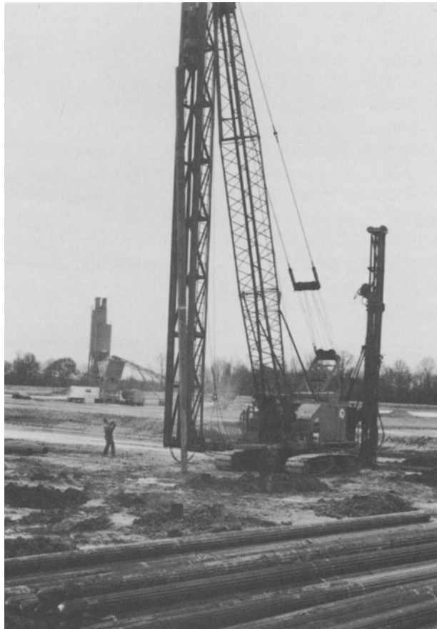
FIGURE 6-3. Installation of steel shell piles. [Ref. 15]
