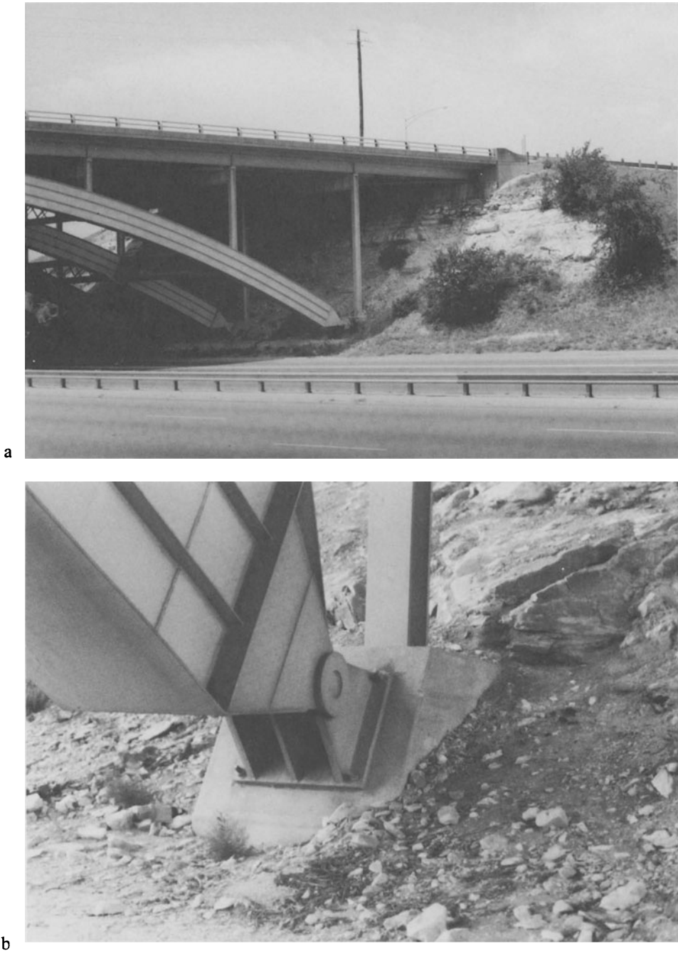
FIGURE 12-2. Arch base bearing on bedrock: (a) overview; (b) close up. [Ref. 21]
