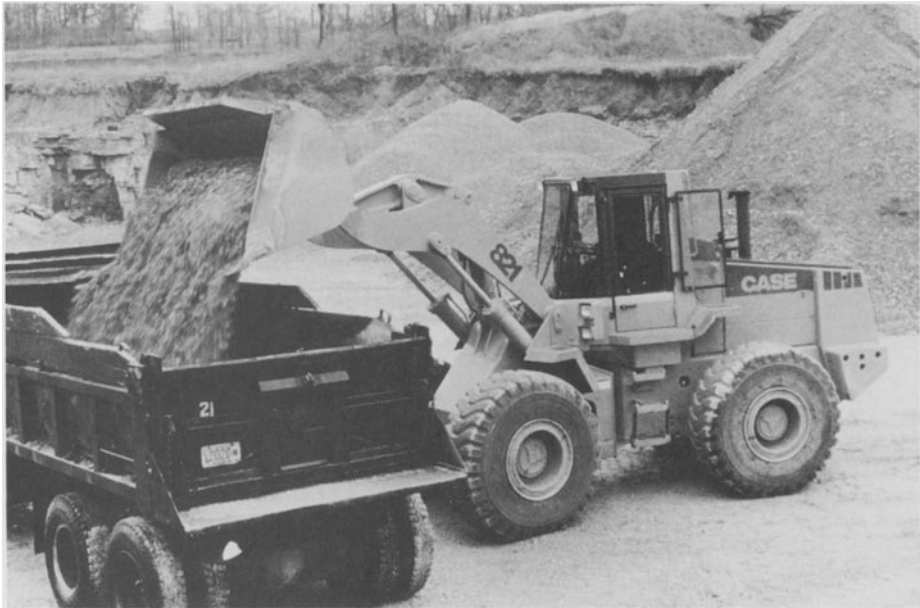
FIGURE 10-1. Soil being loaded at a borrow pit. [Ref. 7]
