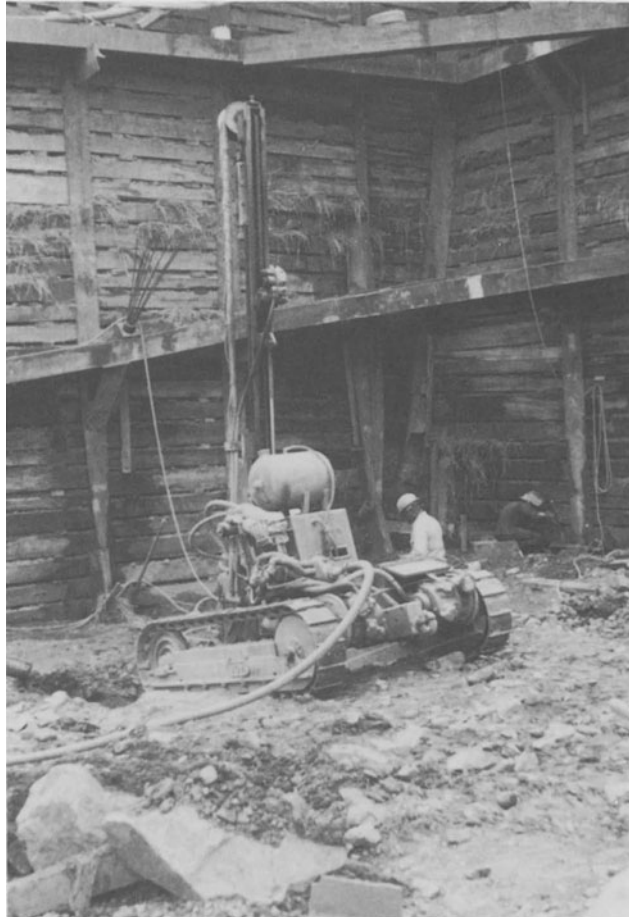
FIGURE 8-19. Rock anchor hole being drilled. [Refs. 9 and 12]
