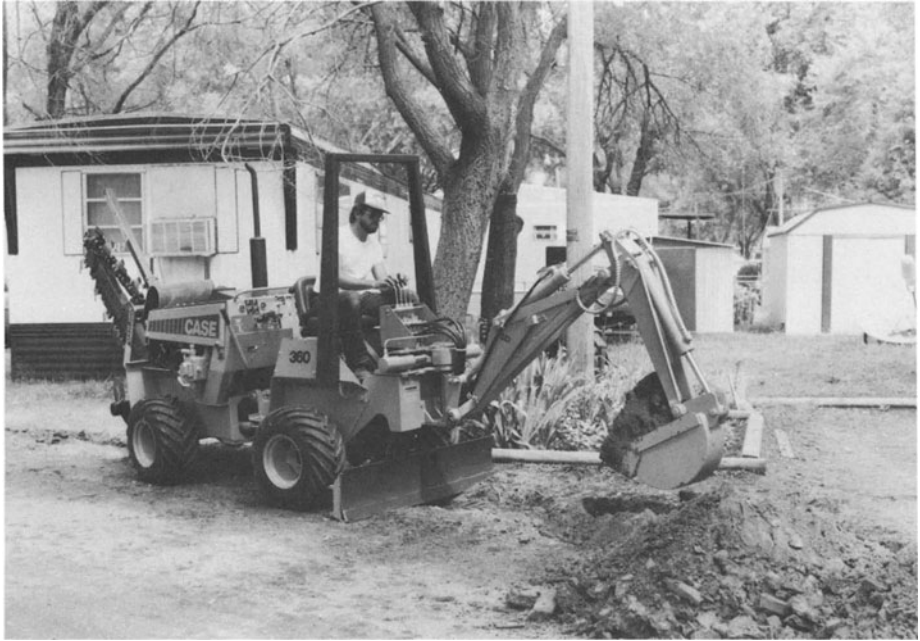
FIGURE 3-2. A backhoe in the process of cutting a trench for visual examination of a soil profile. [Ref. 7]
