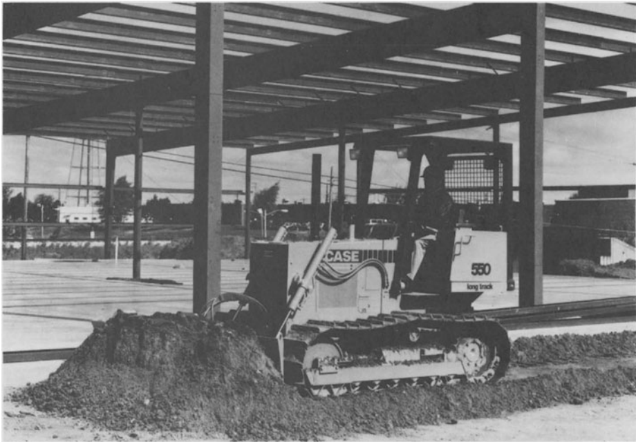
FIGURE 10-2. Spreading soil before compaction. [Ref. 7]
