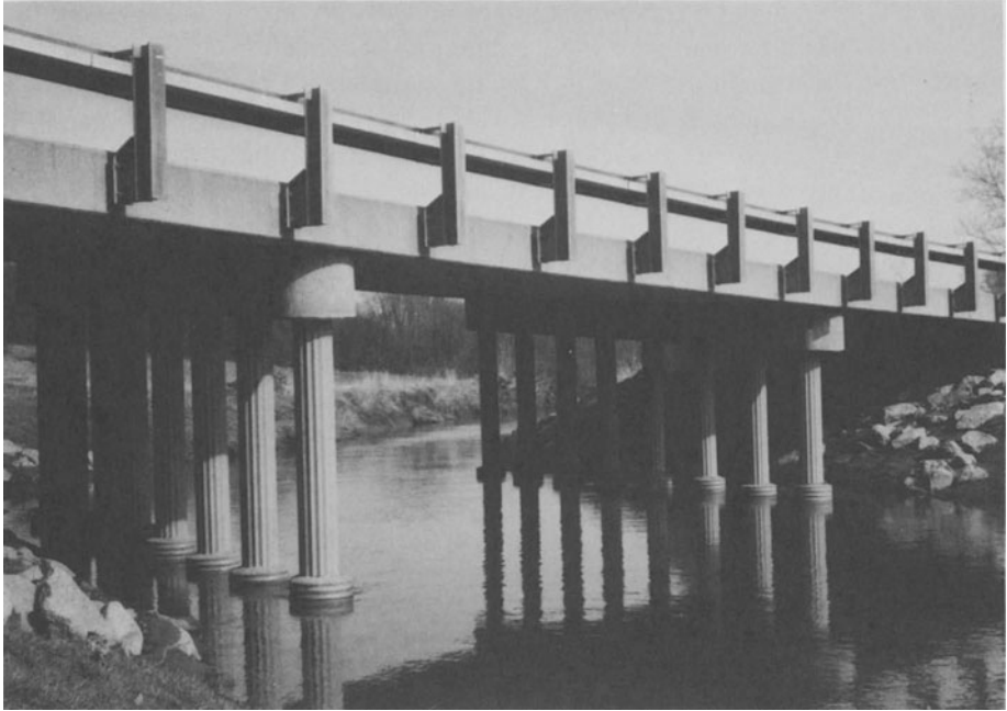
FIGURE 6-4. The aesthetic use of piles. [Ref. 15]
