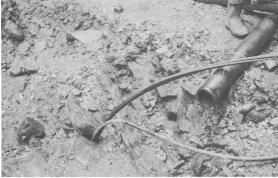
FIGURE 8-20. Rock anchor cable and grout tube positioned in hole prior to grouting the dead end anchorage. [Refs. 9 and 12]
